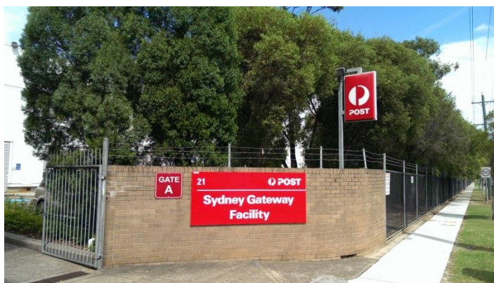
Figure: Australia Post’s Sydney Gateway Facility in Granville
